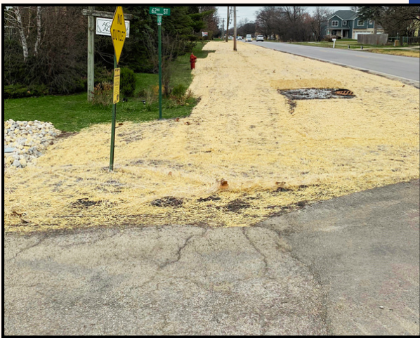
Water Detention Project
