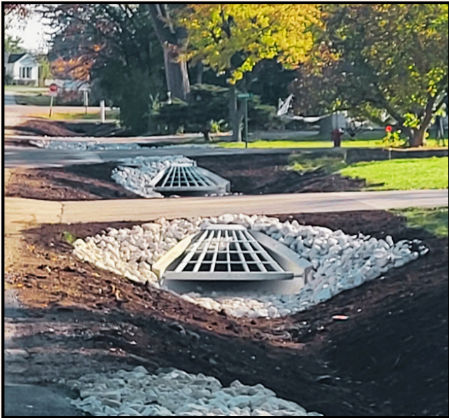
Drainage Project in La Grange Highlands
