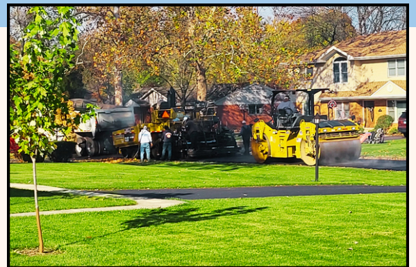
Road resurfacing crew
