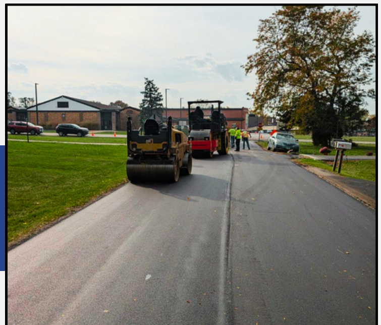
Road resurfacing Howard Avenue
